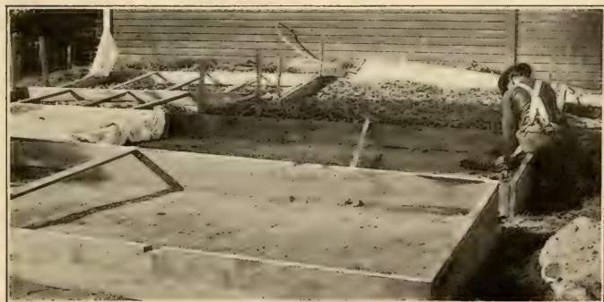
PLATE XIX. — Above , shacks in large strawberry fields, southern California, occupied by the Japanese laborers who rent the land; below , coldframe used as a cutting bed in summer bedding.
